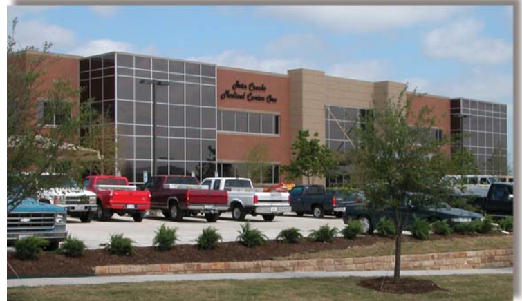
Twin Creeks Medical Center One was completed in May and is leasing quickly. Building Two is planned to begin construction in the fall.
