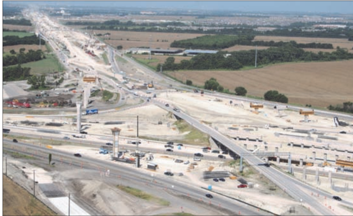
Construction of the Highway 121 / US 75 interchange
